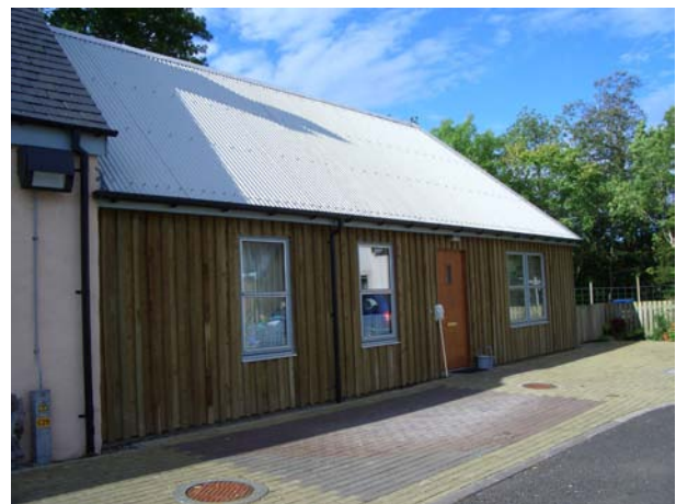
Figure 18.5 The slaughterhouse showing untreated timber cladding.
