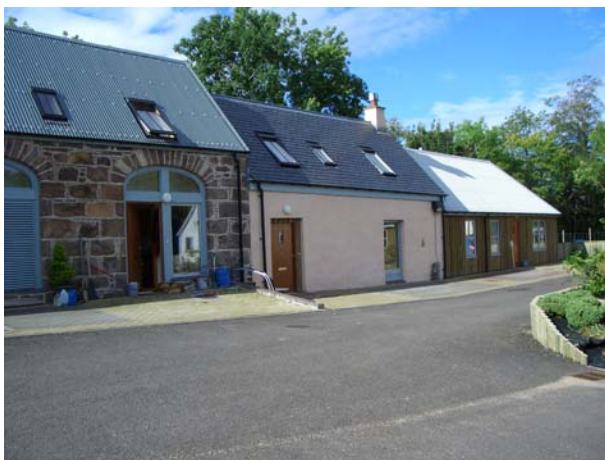
Figure 18.4 Corrugated metal roof for the barn conversion.
